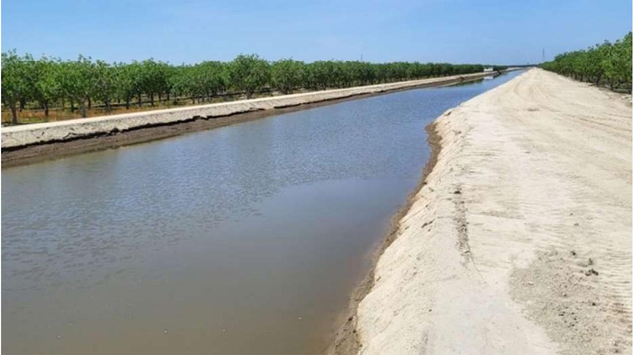
Water in an unlined canal conveyance system with pistachios orchards on either side.
